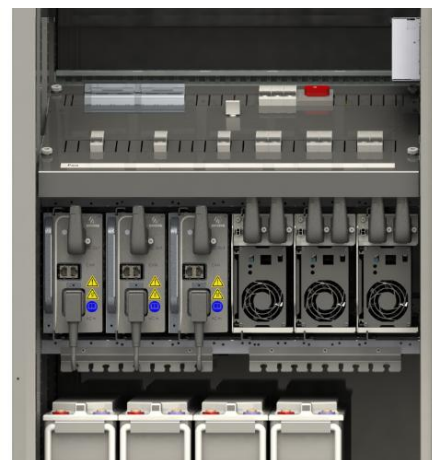
Converters installed to OPUS cabinet
